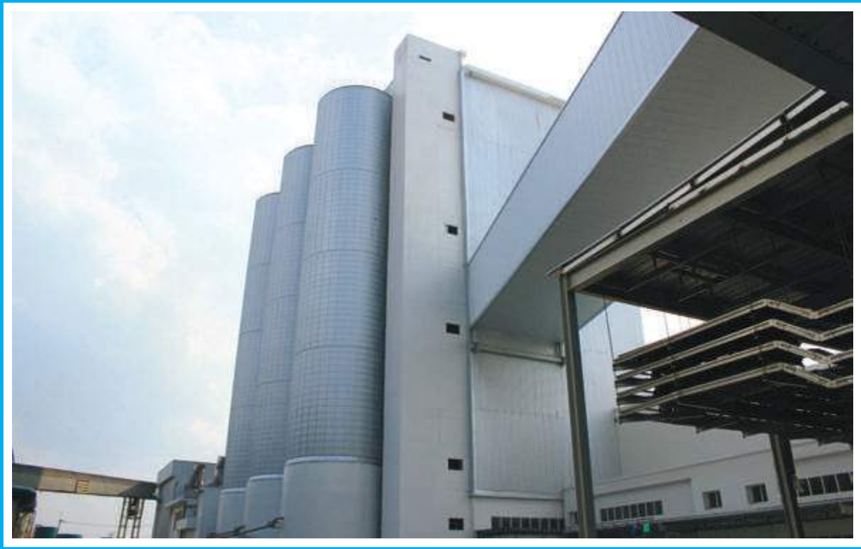
2013 Mitr Phol Refinery Plant and GMP Warehouse, Khonkaen
